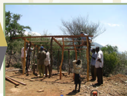
Building a House in Ortum
